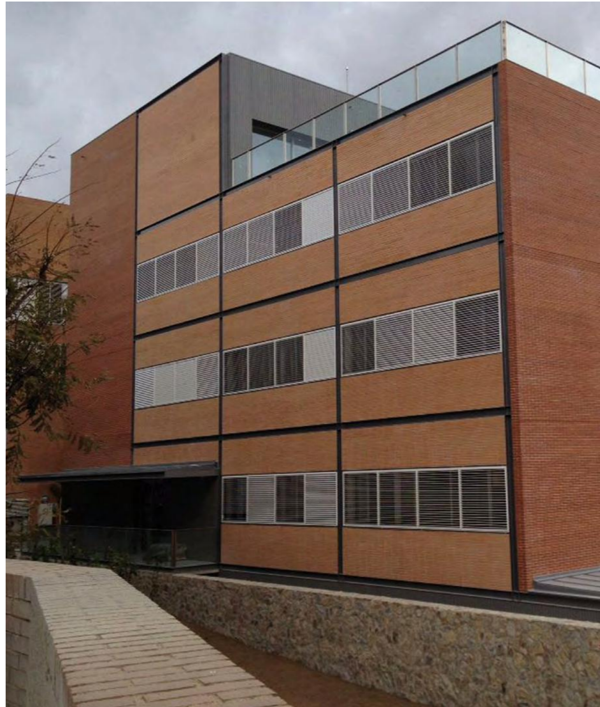
New premises of Flumen Institute at UPC Campus Nord (B0 building)
