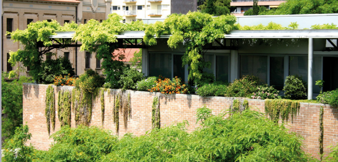
C1 Building at Campus Nord UPC Barcelona
