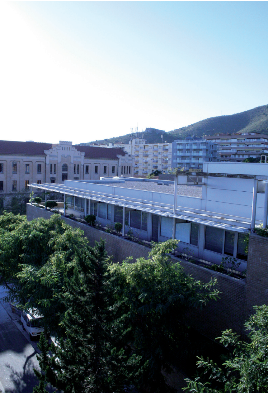
View of CIMNE - Barcelona building
