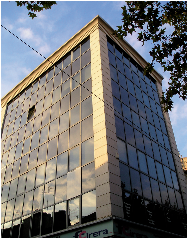
Building housing Bee-Group in Terrassa
