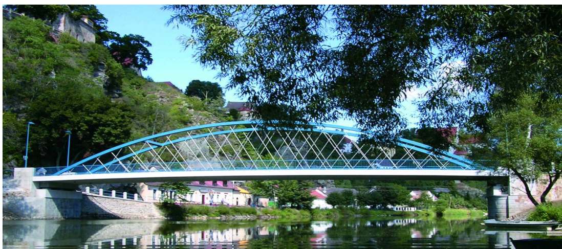
Figure 4. Bridge over the river Lužnice close to Bechyně in the Czech Republic [LIM]
